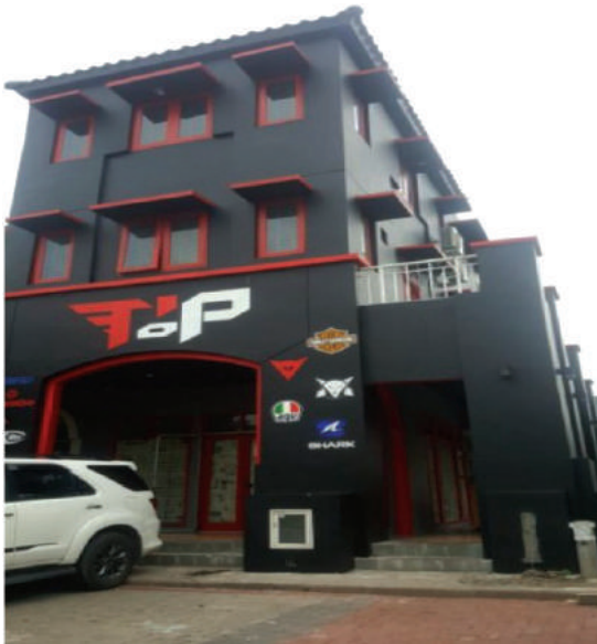
Gambar 2. Tampak Facade Bangunan TIP TOP Apparel & Bike
