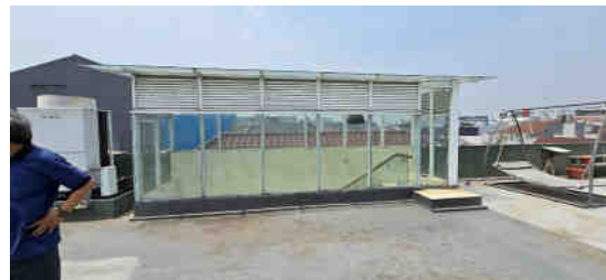
Figure 11. Glass room on the rooftop Source: Author, 2025
