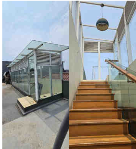
Figure 10. Glass room at the roof top Source: Author, 2025
