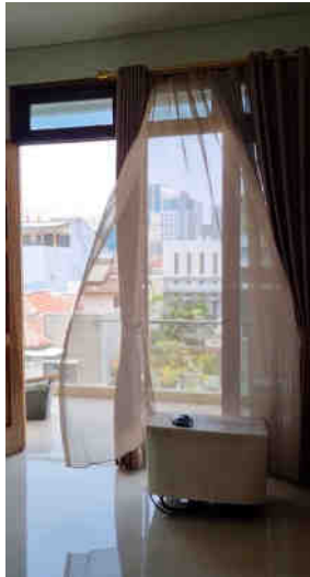
Figure 21. Operable windows used as inlet openings Source: Author, 2025
