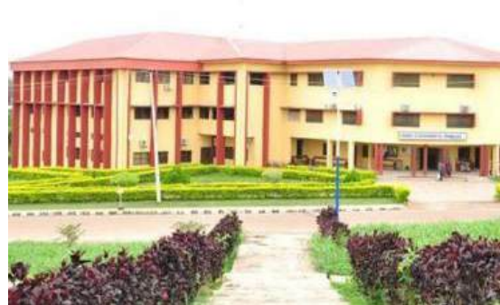
Figure 5. Image of the School of Environmental Technology Building at FUTA. Source: Emaikwu, 2025
